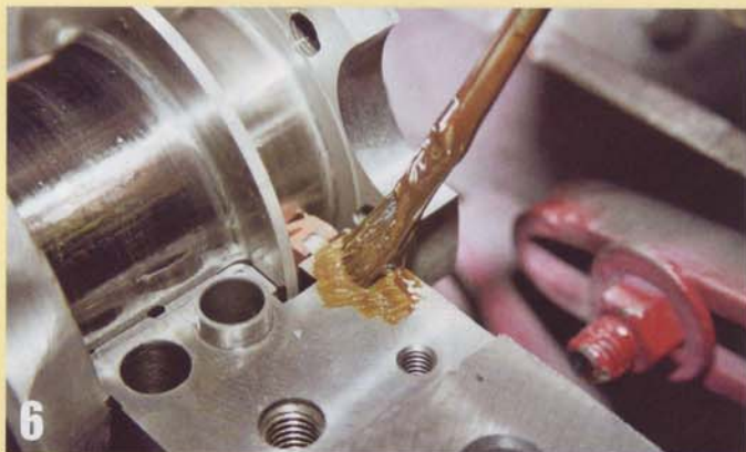
6 Follow the same procedure for installing the seal in the cap. Larry likes to place some sealant on the block where the cap meets the seal.
