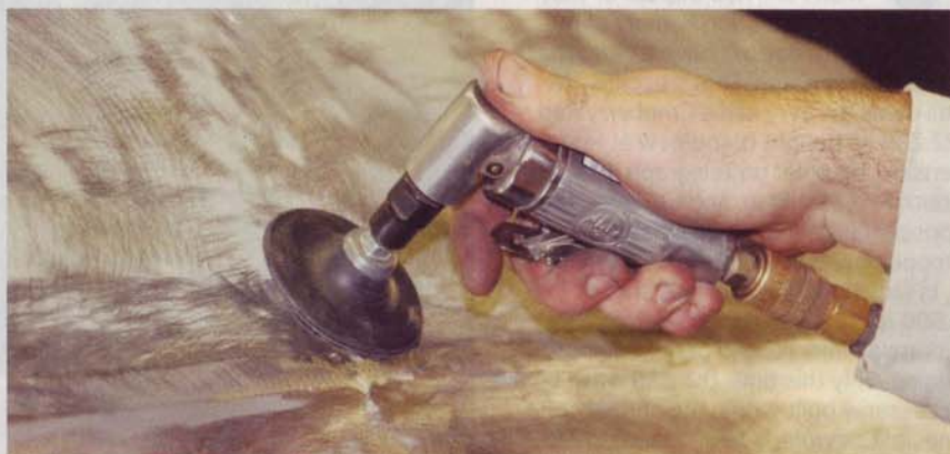
19 When the metal was where it needed to be, the stud was cut off and ground smooth. This method is far superior to drilling holes into panels in order to accomplish the same result.
