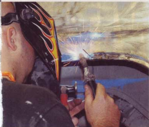
16 Rock welded the metal to the formerly cancerous portion of the wheel lip.
