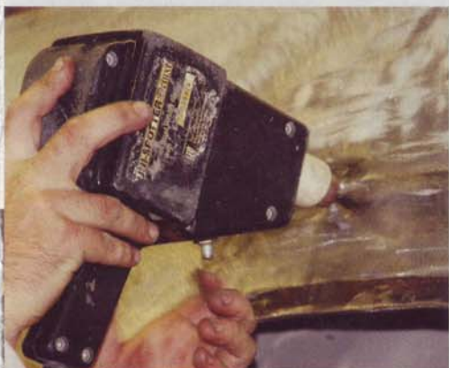
17 An H&S Uni Spotter Delux Stud Welding Gun sent a stud to the quarter at the low point.
